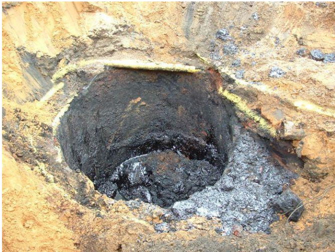
Excavating a circular tar well at a small country gasworks in Norfolk.
